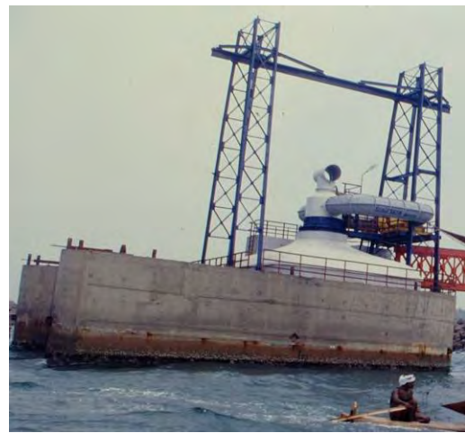
Fig. 2b. The Indian wave energy plant, 1996
