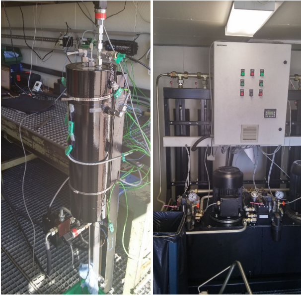
(a) Test Accumulator (b) Hydraulic Supply
