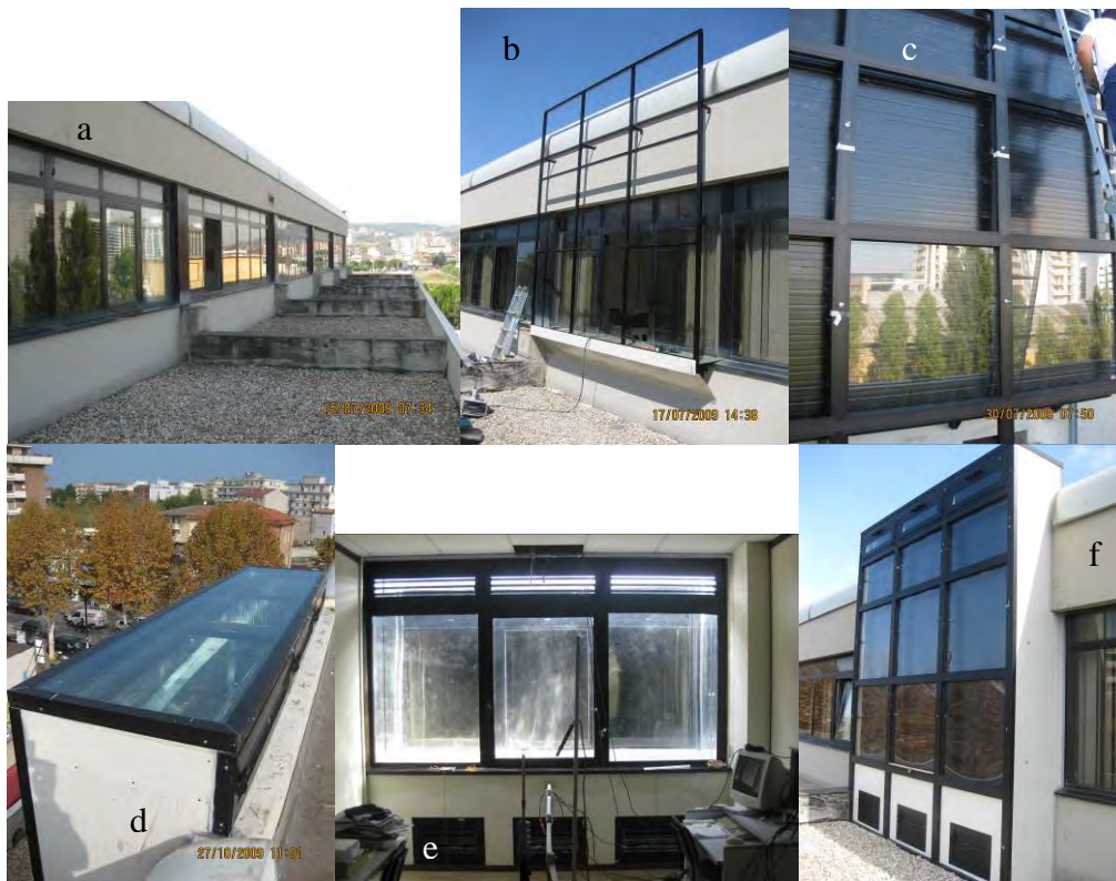
Fig. 1. Realization steps of the VIW.
