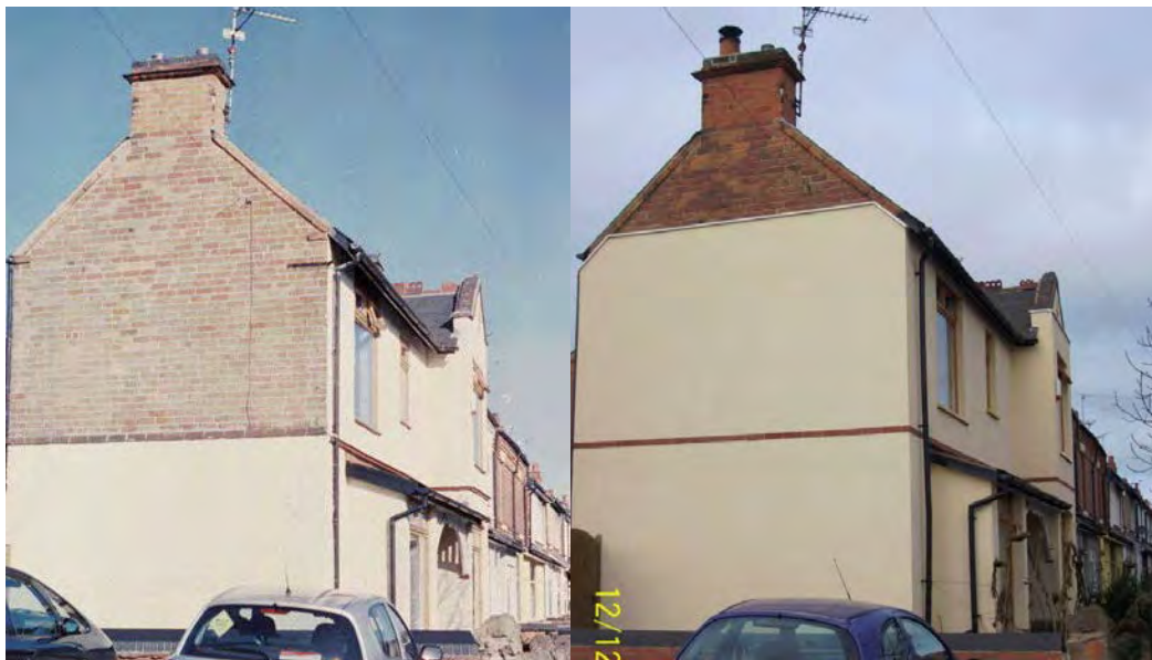
Figure 1. View of house from south side, before and after external insulation.
