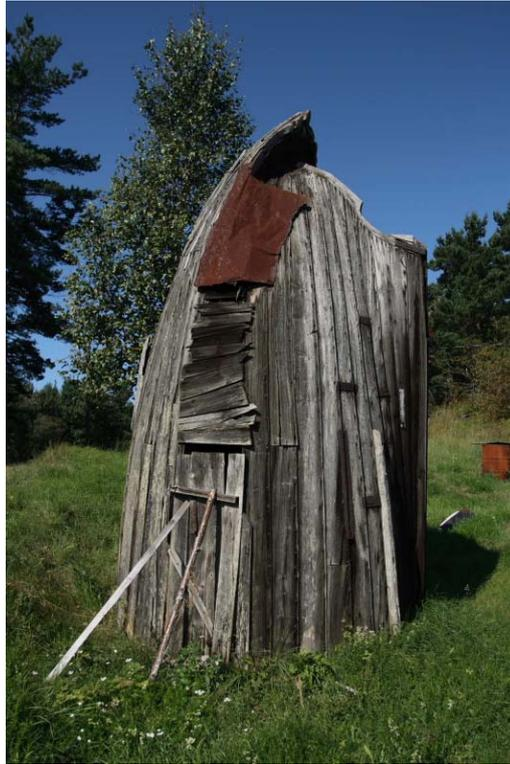
Picture 3: Traditional Liv smoking house made out of a boat cut in half
