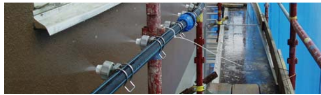
Figure 1. Application of ultra-clean water on the facade by a piping system with nozzles [9].
