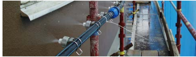
Figure 1. Application of ultra-clean water on the facade by a piping system with nozzles [9].
