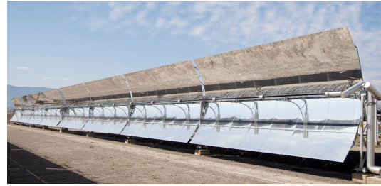
Figure 1. Lateral view of the first TCP-100 PTC in the first loop at Plataforma Solar de Almería (PSA-CIEMAT). It is composed of 8 modules of 12 meters length each.
