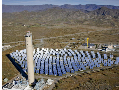
Figure 1. CESA-I central receiver research facility at Plataforma Solar de Almería (PSA).
