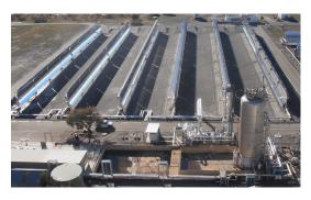
**Figure 2.** Top view of the TCP-100 field at Plataforma Solar de Almería (PSA-CIEMAT). The three loops are shown, with two PTCs in each of them, numbered from 1 (rightmost) to 6 (leftmost). The first loop is formed by the connected pair 1-2 (right loop), the second loop by 3-4 (center loop) and the third by 5-6 (left loop).
